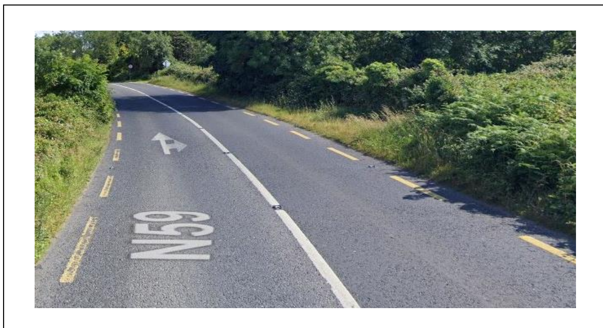
Figure 4.2: Hidden Dip on approach to junction from Moycullen direction (West)
